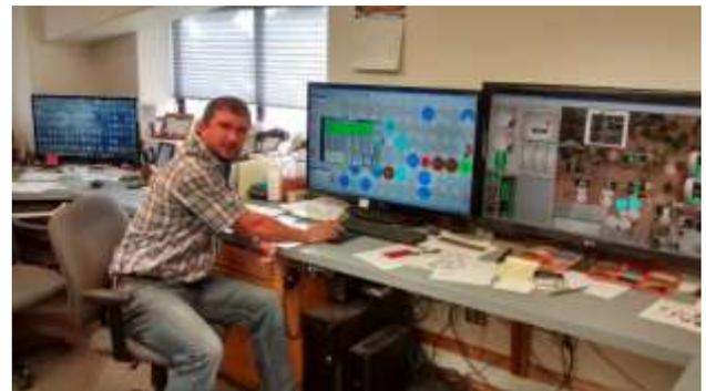
Figure 4. Information about water and power use is relayed via the internet. The system can be monitored and adjusted from the office or elsewhere in real time. Photo: Erin Brooks.
